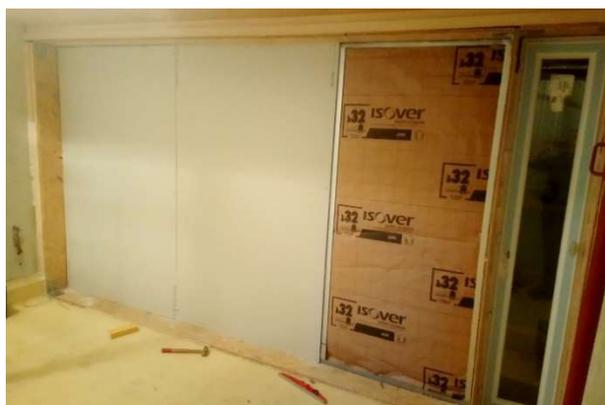
**Fig. 2.** Photography of the wall (without one gypsum board)
