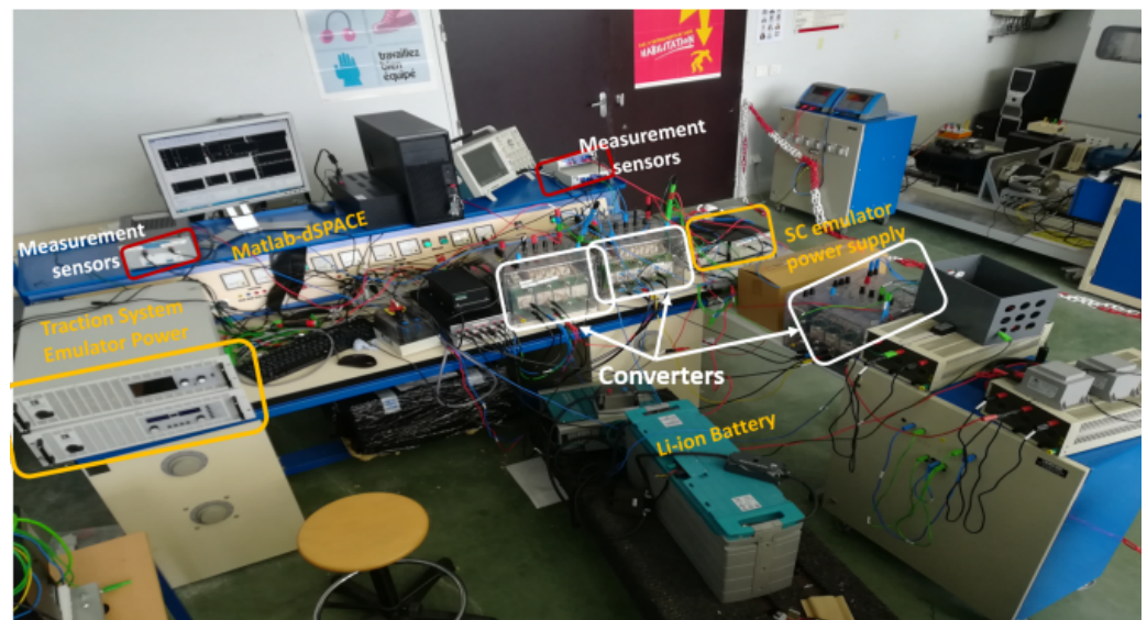
Figure 9. Experiment test bench in S2ET-Lab in ESTACA-LAVAL.
